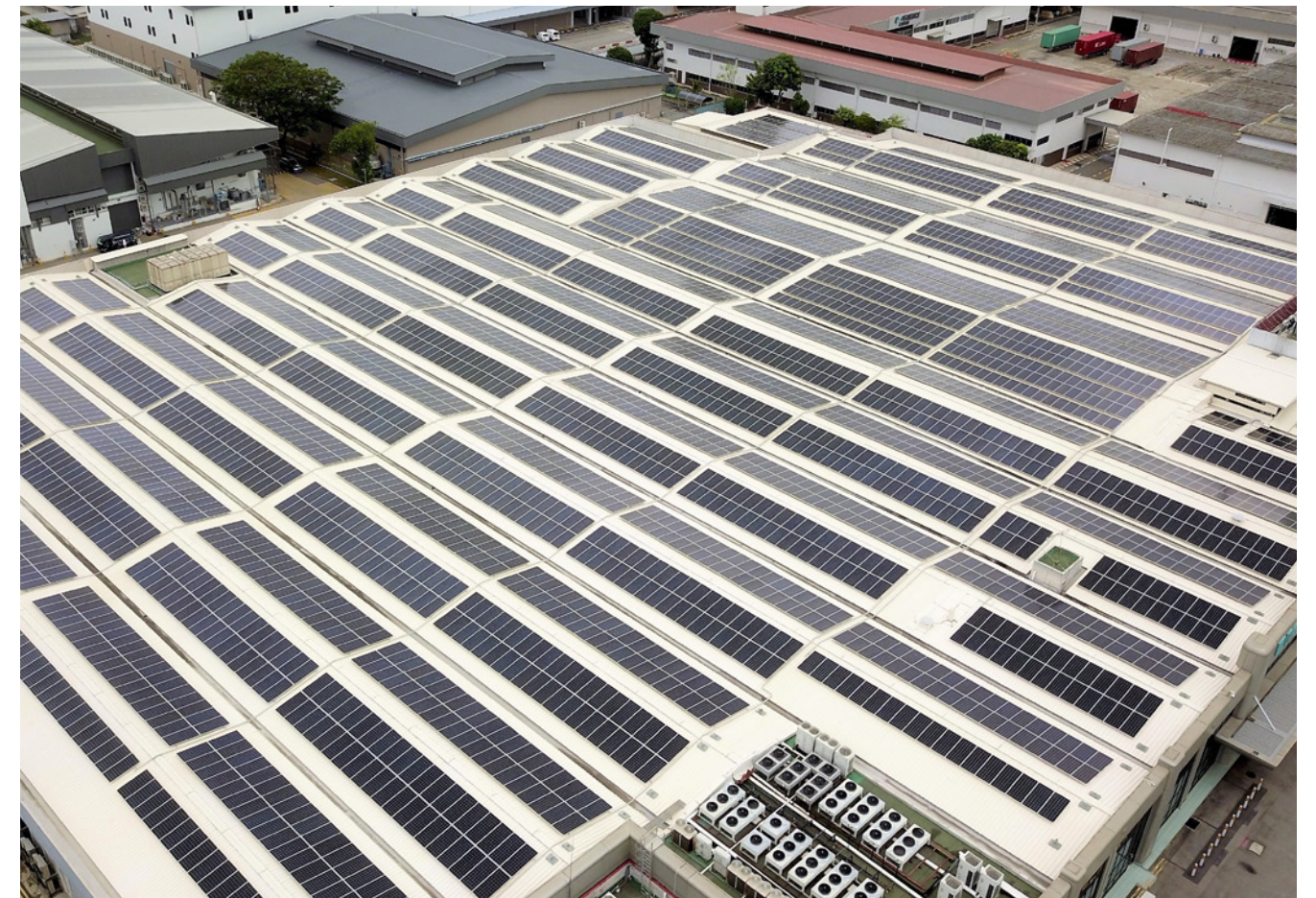
Solar panels on the rooftop of NCS Bedok Data Centre
